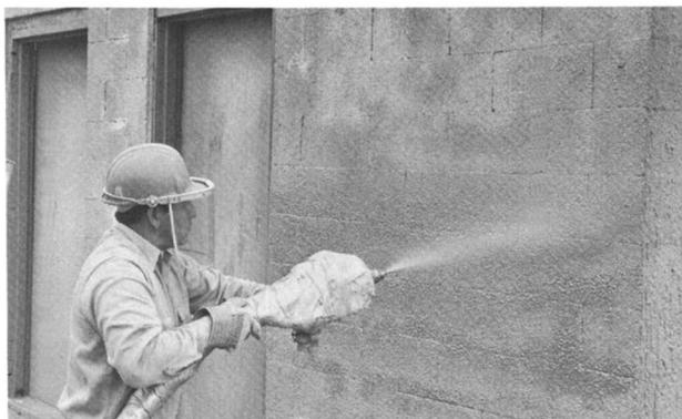
*Figure 6. Spraying the sulfur formulation on the cinder block walls*
