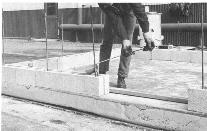
*Figure 1. Bonding the first course of block to the concrete slab*
