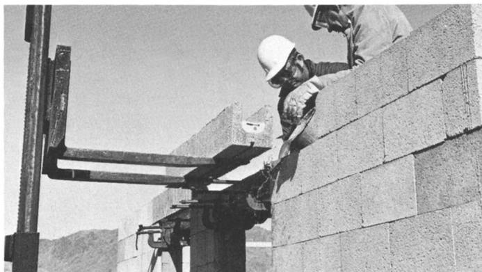
*Figure 5. Inserting lintel beam over a door opening*
