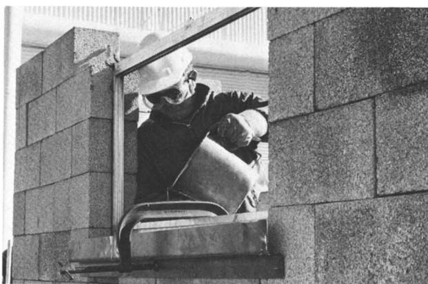
*Figure 2 (top). Dry-stacking the block to build the walls. Figure 3 (middle). Grouting the steel door frames to the block with the sulfur formulation. Figure 4 (bottom). Forming the window sill with the sulfur formulation.*
