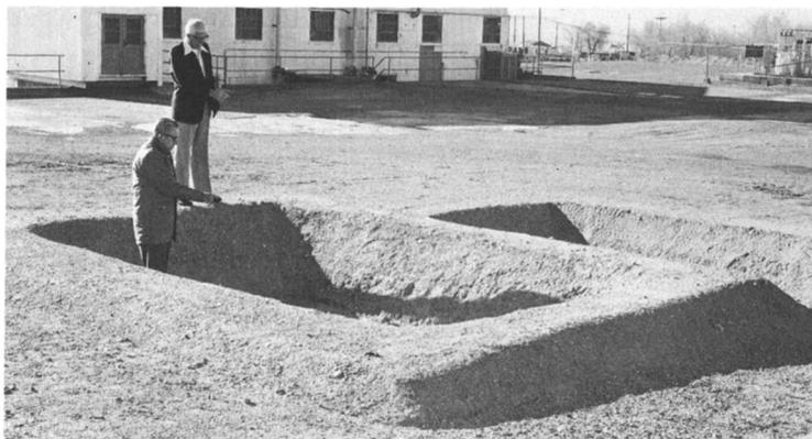
**Figure 9. Excavated form for the double pond**
